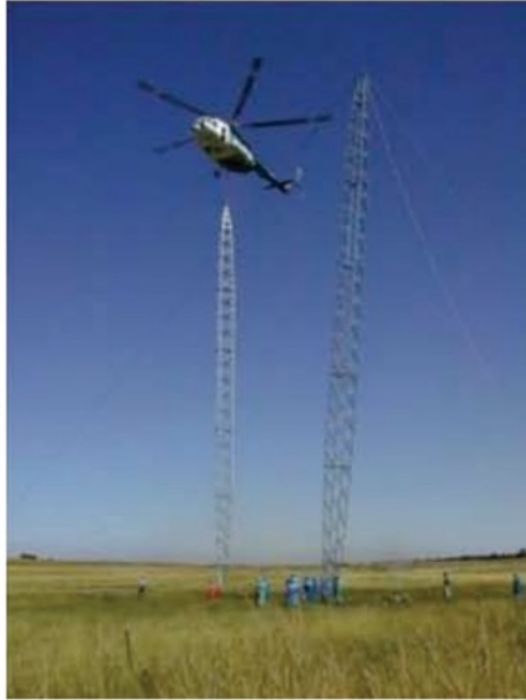
Figure 3: Typical construction equipment
